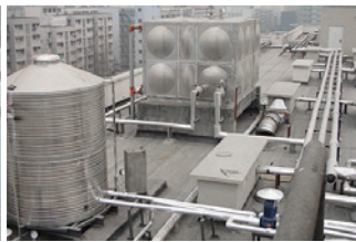
Water tank fabrication
